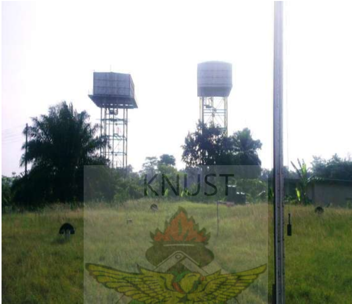
Figure 3.2 KNUST overhead tanks (250 cubic metres each)
