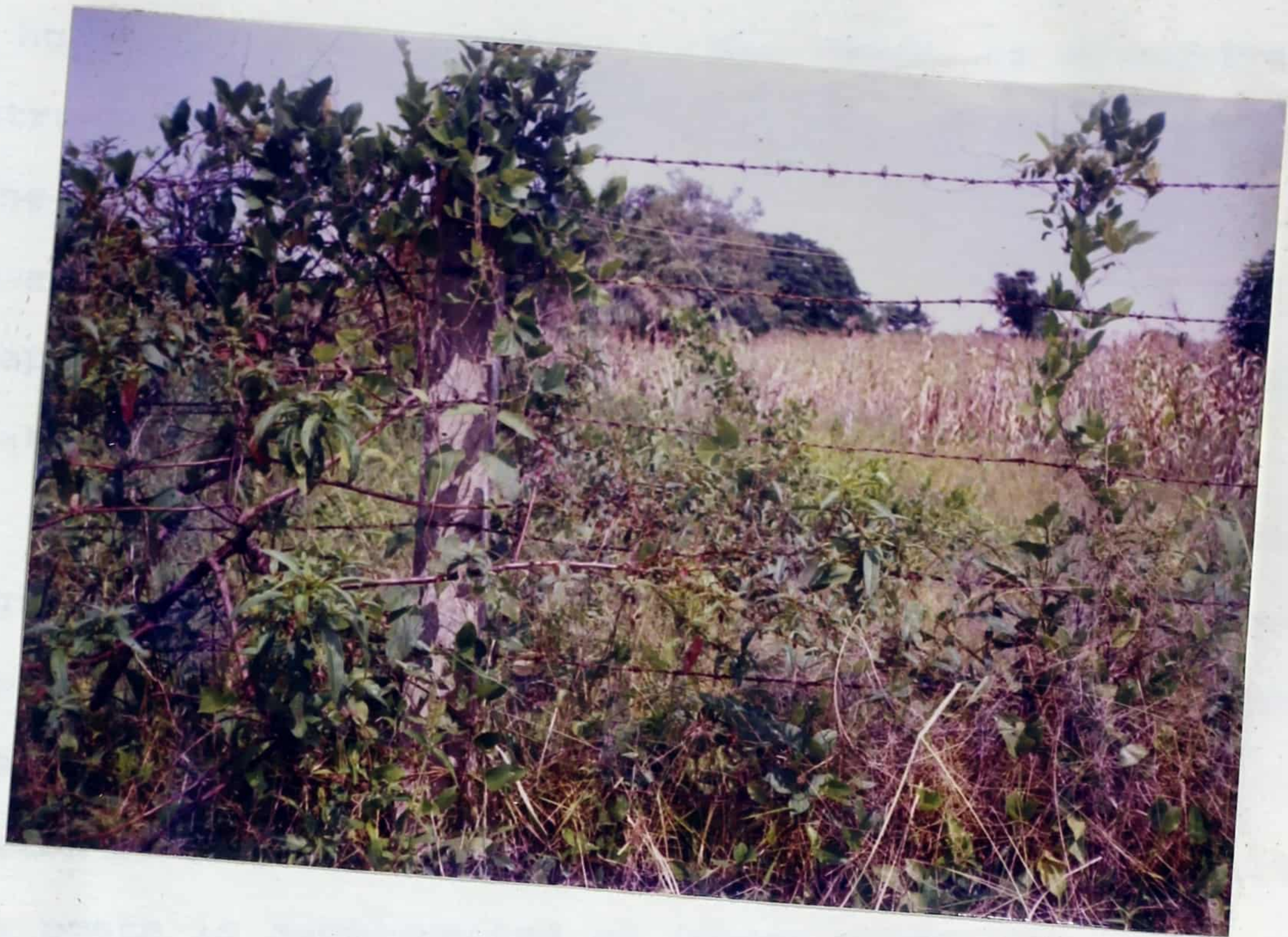
Plate 24: Conventional concrete fence posts with wire railing at the U.S.T., Kumasi. 1992.
