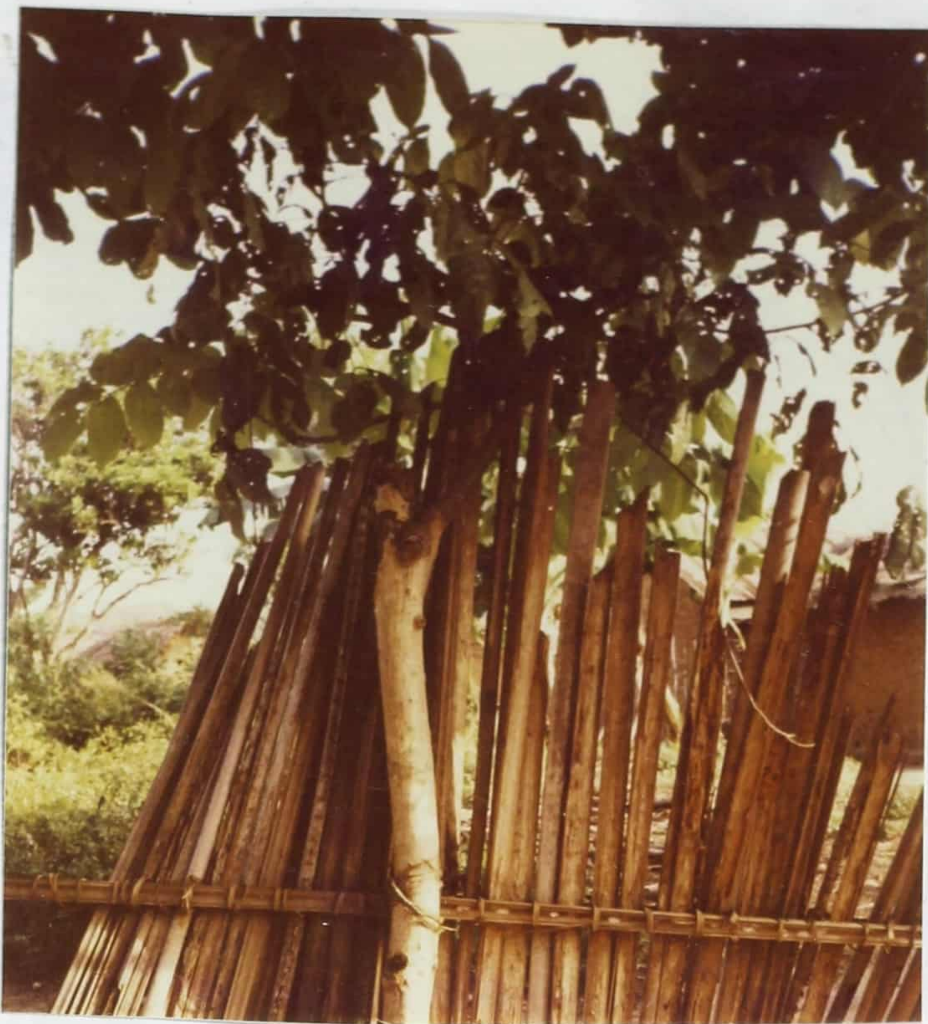
Plate 19: Lannea welwitschii live fence post supporting Raphia battens at the FORIG Guest House, Akotaa. 1992.
