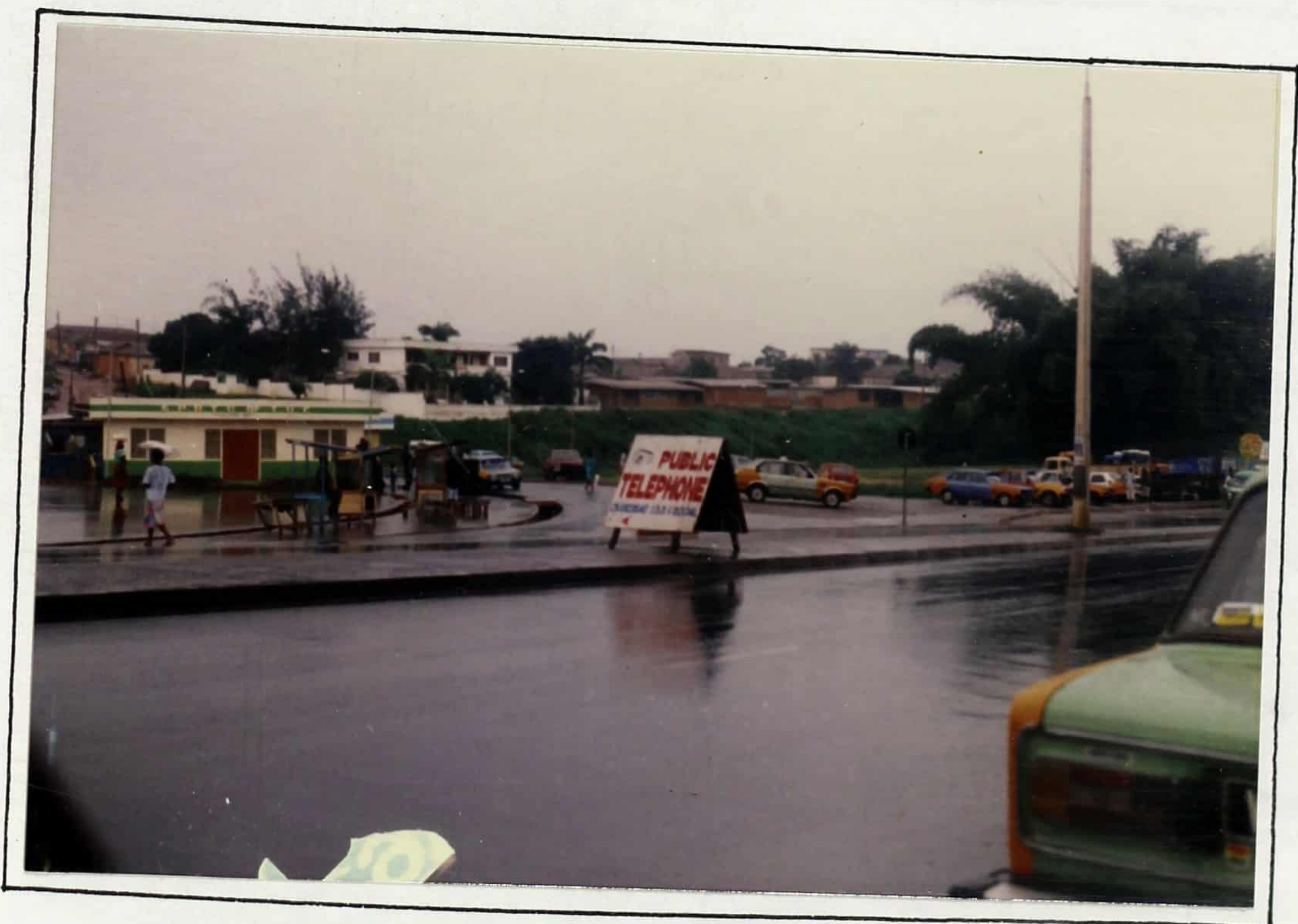
Fig.34. A Signboard Directing People to a Telephone Booth.
